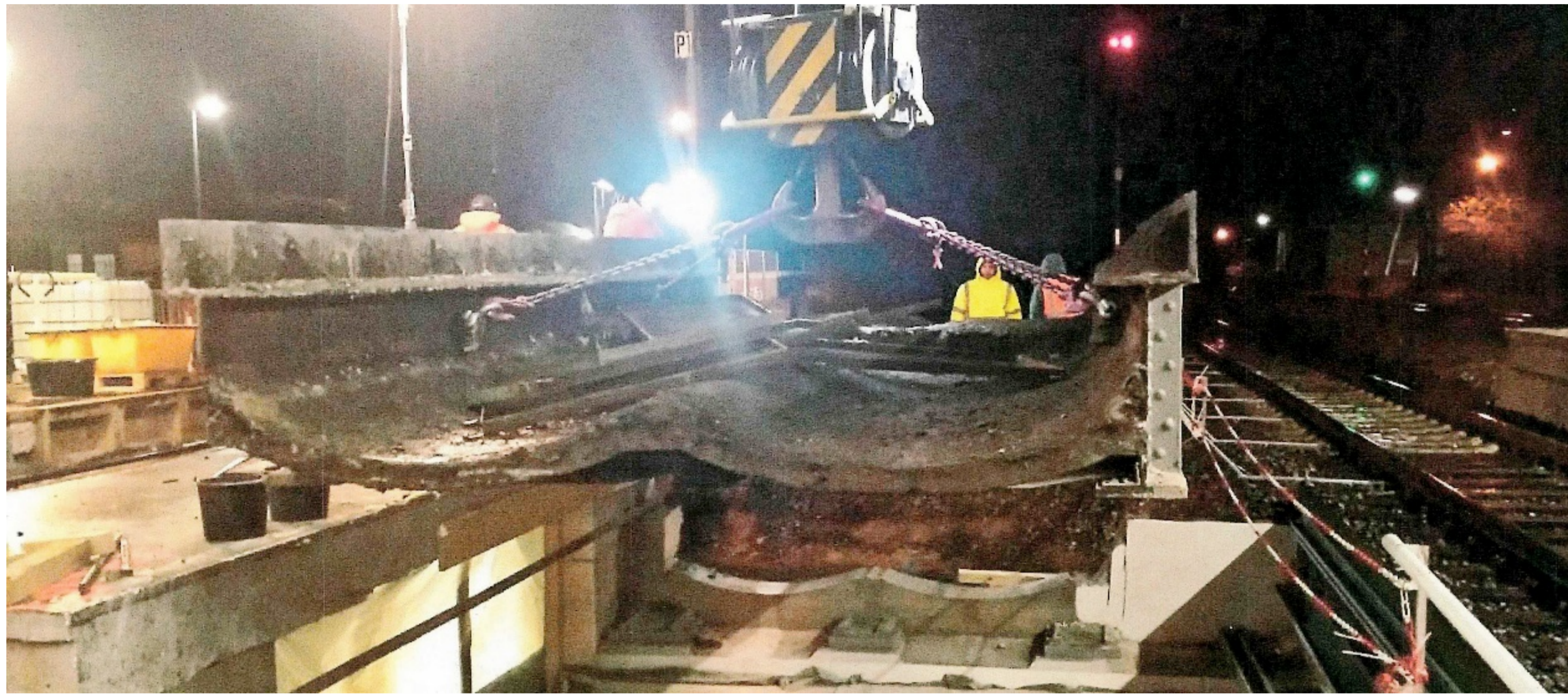
Railroad underpass during dismantling 2020
